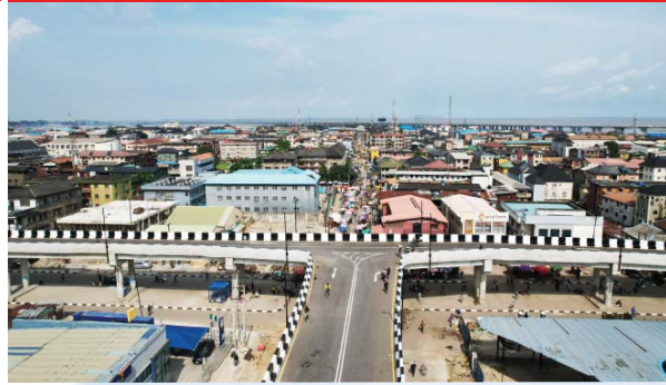
OYINGBO OVERPASS BRIDGE
