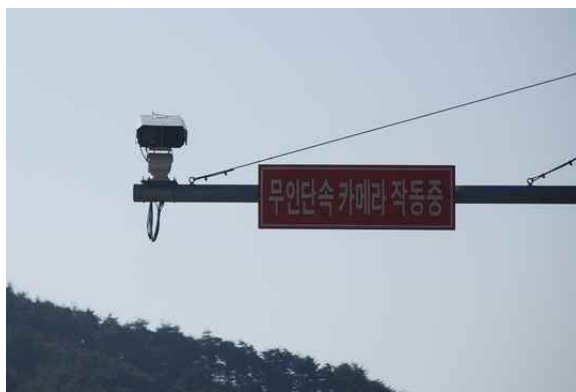
[Figure 4.1-13] Example of installing an automated traffic enforcement camera
