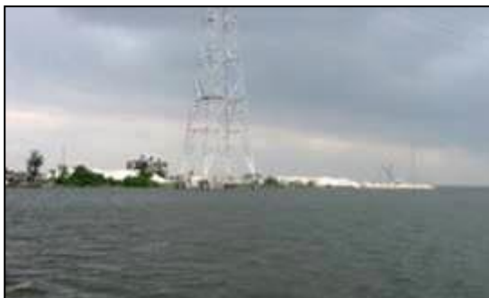
Figure 6.7 – Towers for High Voltage Power Cables on the Lagoon
