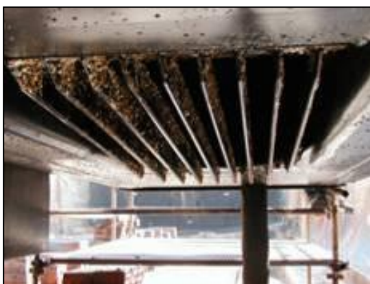
Figure 6.52 – Intake Screens to minimize Inflow of Debris for Water-jets
