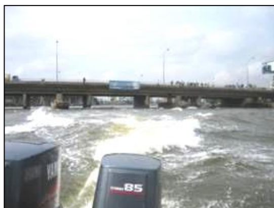
Bridge at Entrance to Five Cowry Creek
